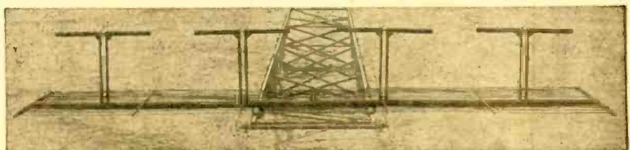
Photo B—A simple horizontal four-element colinear array with a wire-screen reflector.
